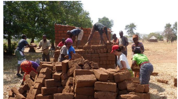
Putting bricks to burn in Nkomba
