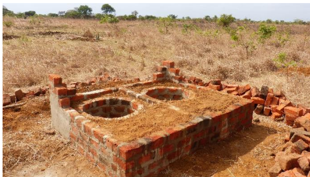
1x2 toilet under construction in Katinti
