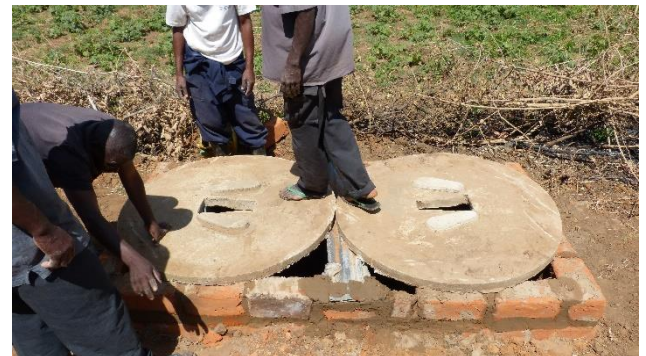
Placing san plates in Kubota
